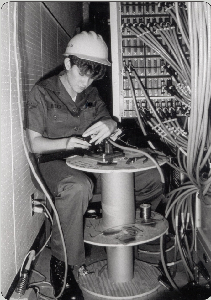
Sharnee Riley, 1837th Engineering Installation Squadron, uses an Amphanol "Amp-Champ" crimper to terminate a connector on one of the multitude of 25-pair cables installed at the control site as part of the Scope Signal III installation to modernize Giant Talk, the Strategic Air Command's world-wide command and controls network, Clark AB, Philippines.
