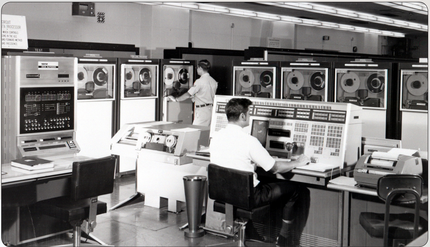
Interior view of the McClellan AFB, California, AUTODIN Switching Center.
